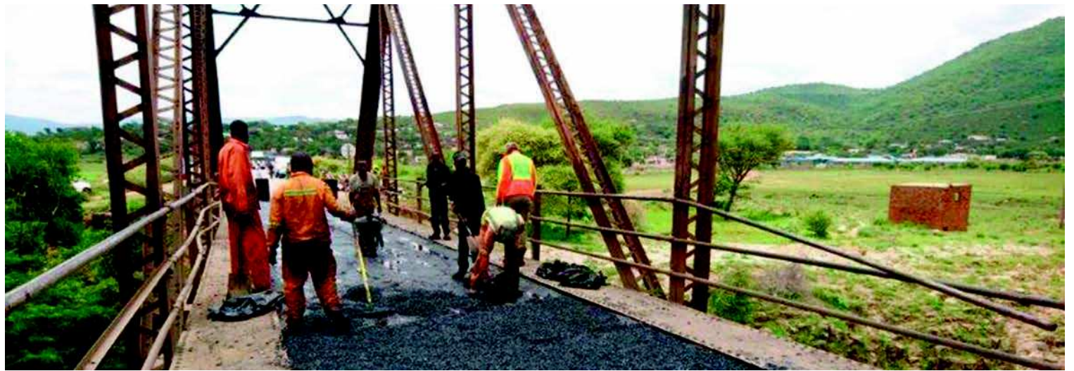
TRP decided to help government maintain some of the local roads.
